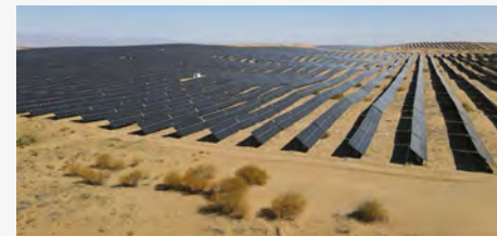
On-site image of 2GW PV-Hydrogen Sand Control Project in Kubuqi Desert, Inner Mongolia
