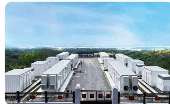
> 25MW/50MWh Generator-side energy storage project in Ledong county, Hainan province
