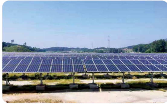
> South Korea 12MW/36MWh Photovoltaic Energy Storage Project
