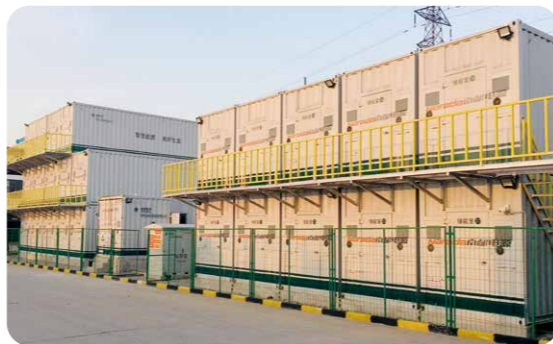
> Jiangsu Jiangnan 6MW/48MWh Chemical Distributed Energy Storage Power Station
